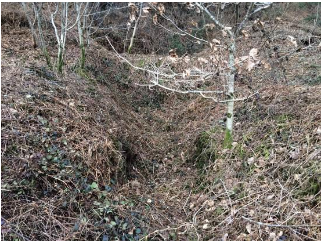
Photograph 27 – Location of adit ref: 276208-040
