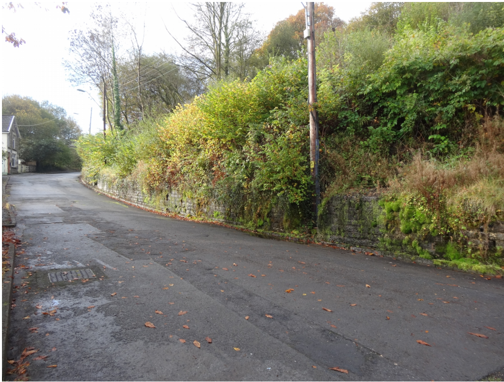
Plate 1: View from Church Road and Graig Road, at the base of Church Road drainage system
